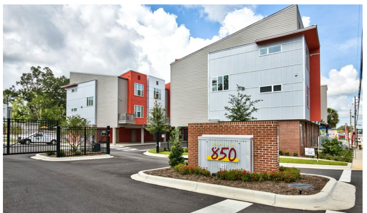
Pictured from top to bottom: Weston Park, a transit-oriented development adjacent to a commuter rail station in Longwood, Florida; Granite Crossing, an affordable family housing community in Lithonia, Georgia; and Arrive 850, a student housing community in Tallahassee, Florida.
