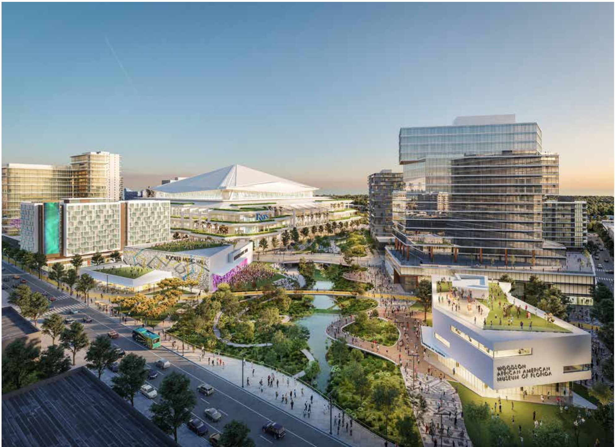
Aerial view of the project looking south along Booker Creek, with First Avenue South in foreground
