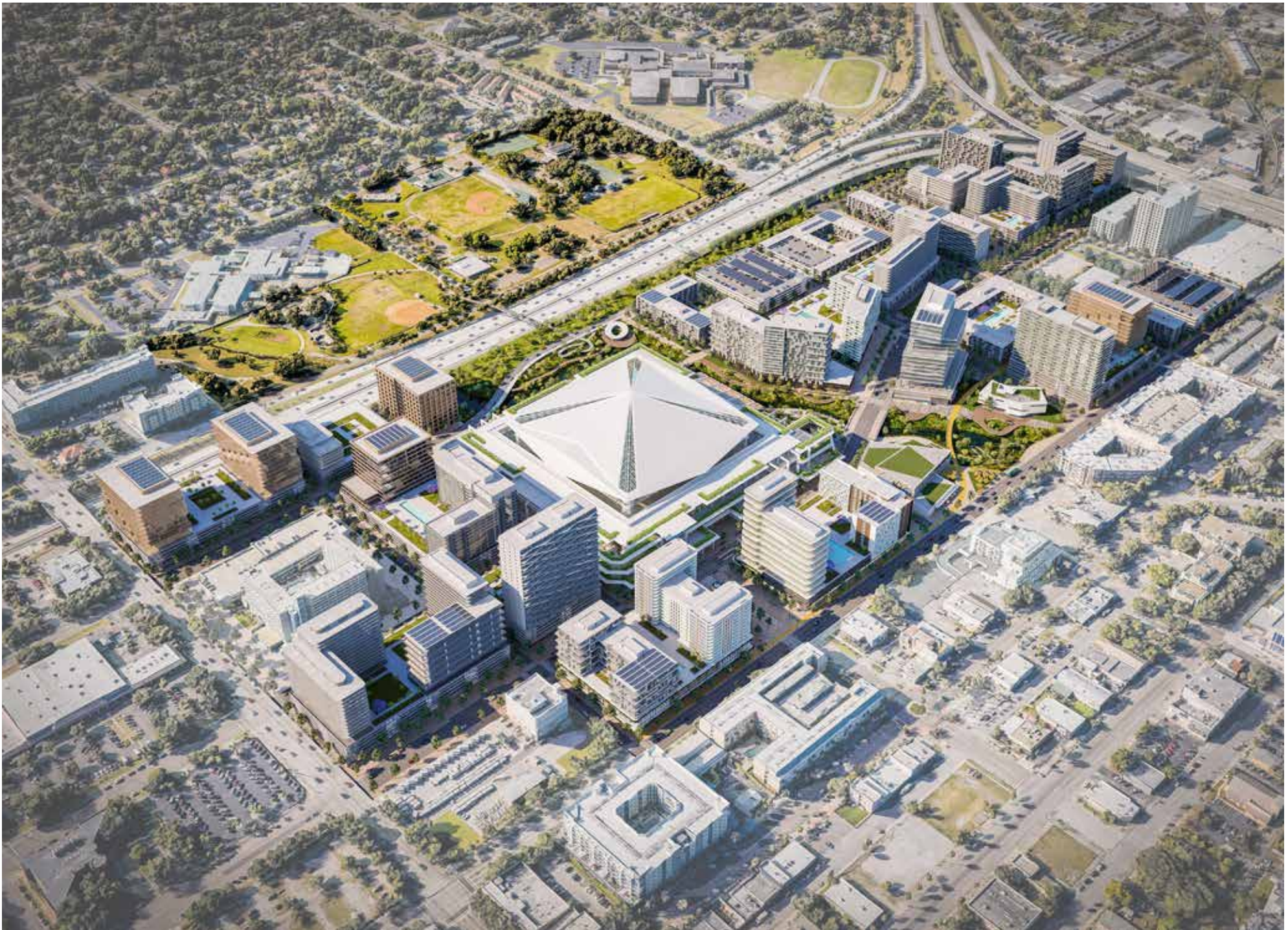
Aerial view of the project looking southwest
