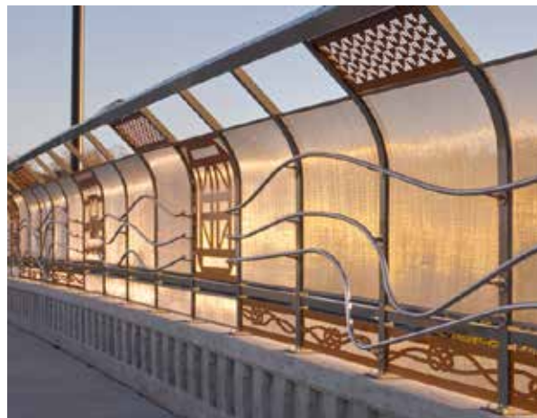
Bridge Cladding as public art; 28th - 31st Avenue Connector, Nashville, TN
