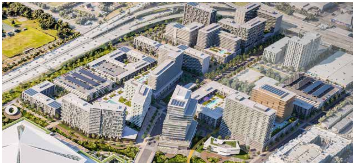
Aerial view of the project west of the Ballpark
